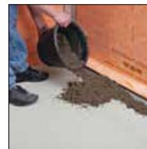
Fig. 3. Apply levelling screed
