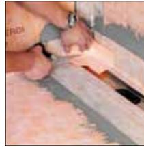
For 2. Adhere KERDI collar/ cut KERECK internal corner to size
